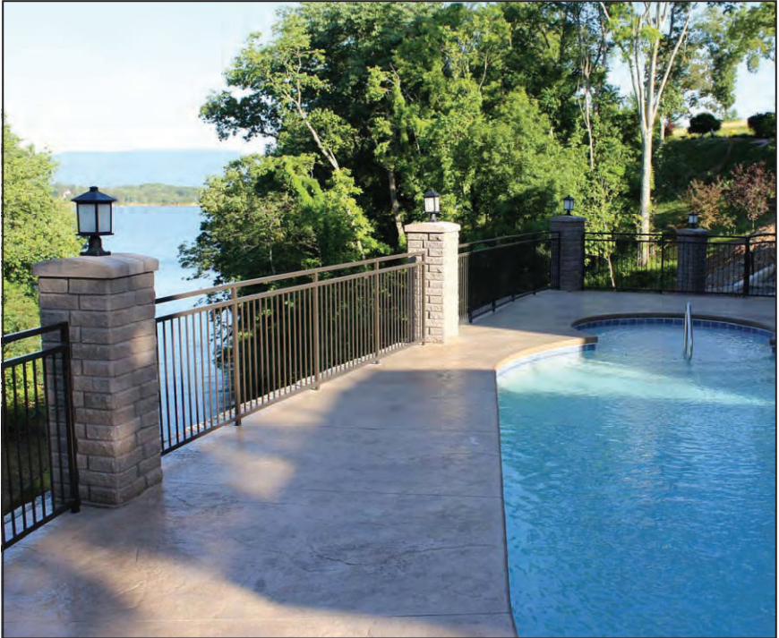
Free Standing Columns
