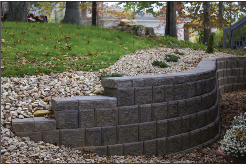
Finished EverLoc® Wall
