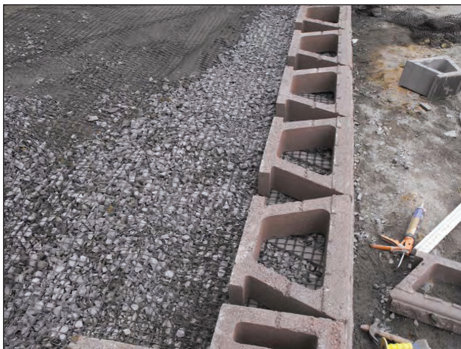
Drainage Aggregate (Inside and behind units)
