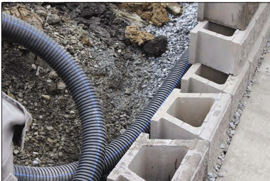
Drainage Pipe Placement
