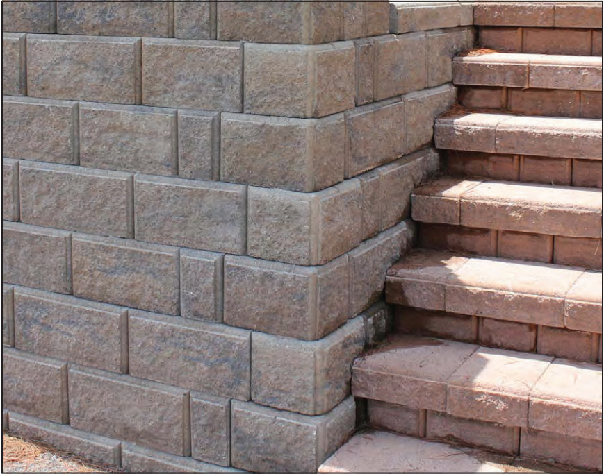
Corner with Utility
